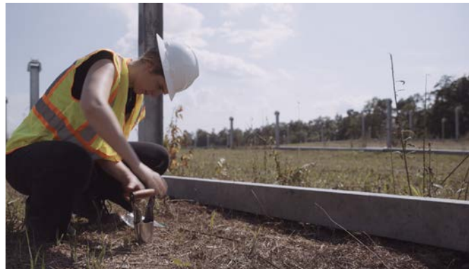
Soil testing underway at the solar project site. Photo: AES
